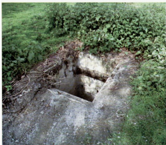
The entrance shaft. When in use there would have been a camouflaged hinged hatch covering the shaft.
